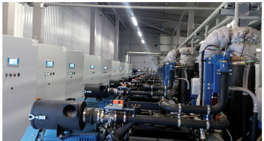
Figure 12. Woodchips cogeneration plant to produce electricity and heat. This plant includes 10 x 45 kW biomass gasifier & CHP installed in the city of Jaunjelgava, Latvia. Ten independent units generate 450 kW of electrical power and 1.08 MW of thermal power. The plants in Jaunjelgava provide a school, a kindergarten and several blocks of flats with heat at 2 ct/kWh. The electricity produced is fed into the national grid at 14 ct/kWh. The total investment was 4700 €/kW e . The charcoal which accumulates during gasification is collected in big bags and sold to Poland.
