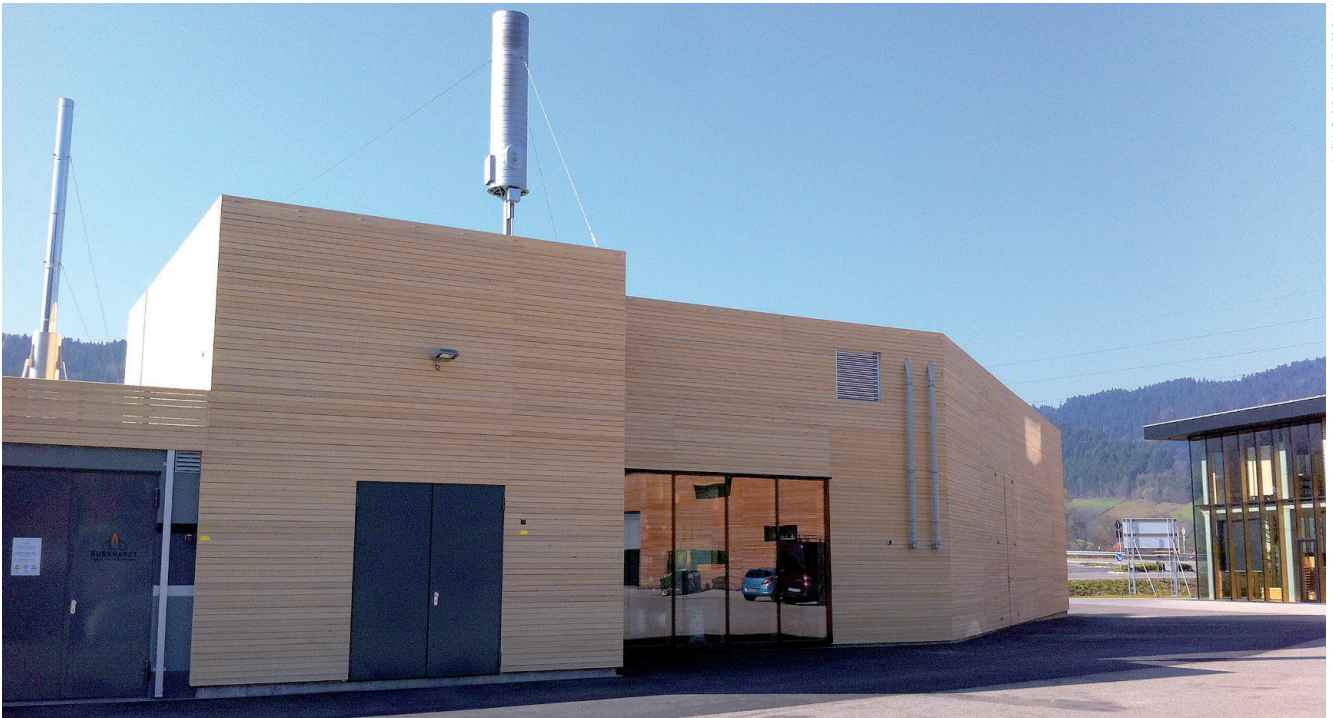
Figure 10. The central element of the plant in Haslach im Kinzigtal, Germany is the biomass gasifier (270kWth/190kWe). The plant is run by Bioenergie Schnelligen. In contrast to what is described in the chapter about Fluidized bed gasification, the plant constructor Burkardt has turned the process upside down: The fuel is fed into the reactor from below. The reactor is served by high quality pellets from the region and can serve 400 households including local heating for window construction company, paint shop, gardening, a hotel with spa and several single houses with heat and electricity is fed into the grid. In addition this plant also has a natural gas CHP system (248kW th /210kW e ).
